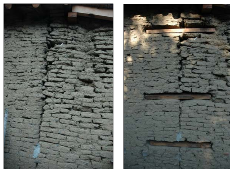
Insertion of wooden beams to "tie" and strengthen mud brick walls
