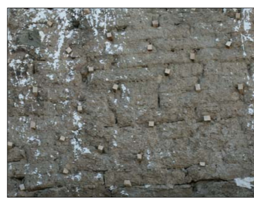
Wooden pegs to receive new plaster
