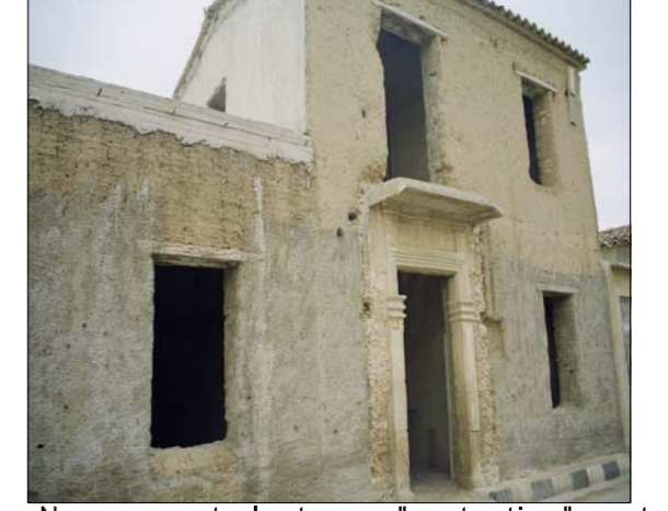
New cement plaster as "protective" coat
