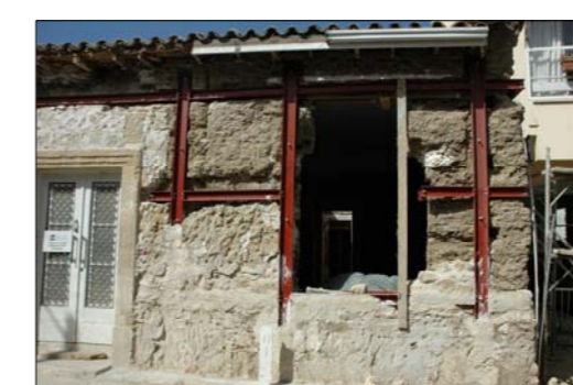
New metallic structure inserted into mud brick wall
