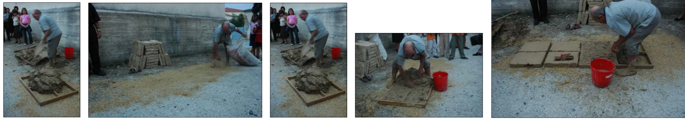
Mud brick construction
