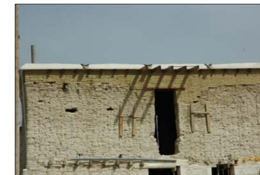
Completion of missing upper part of the wall with new adobe
